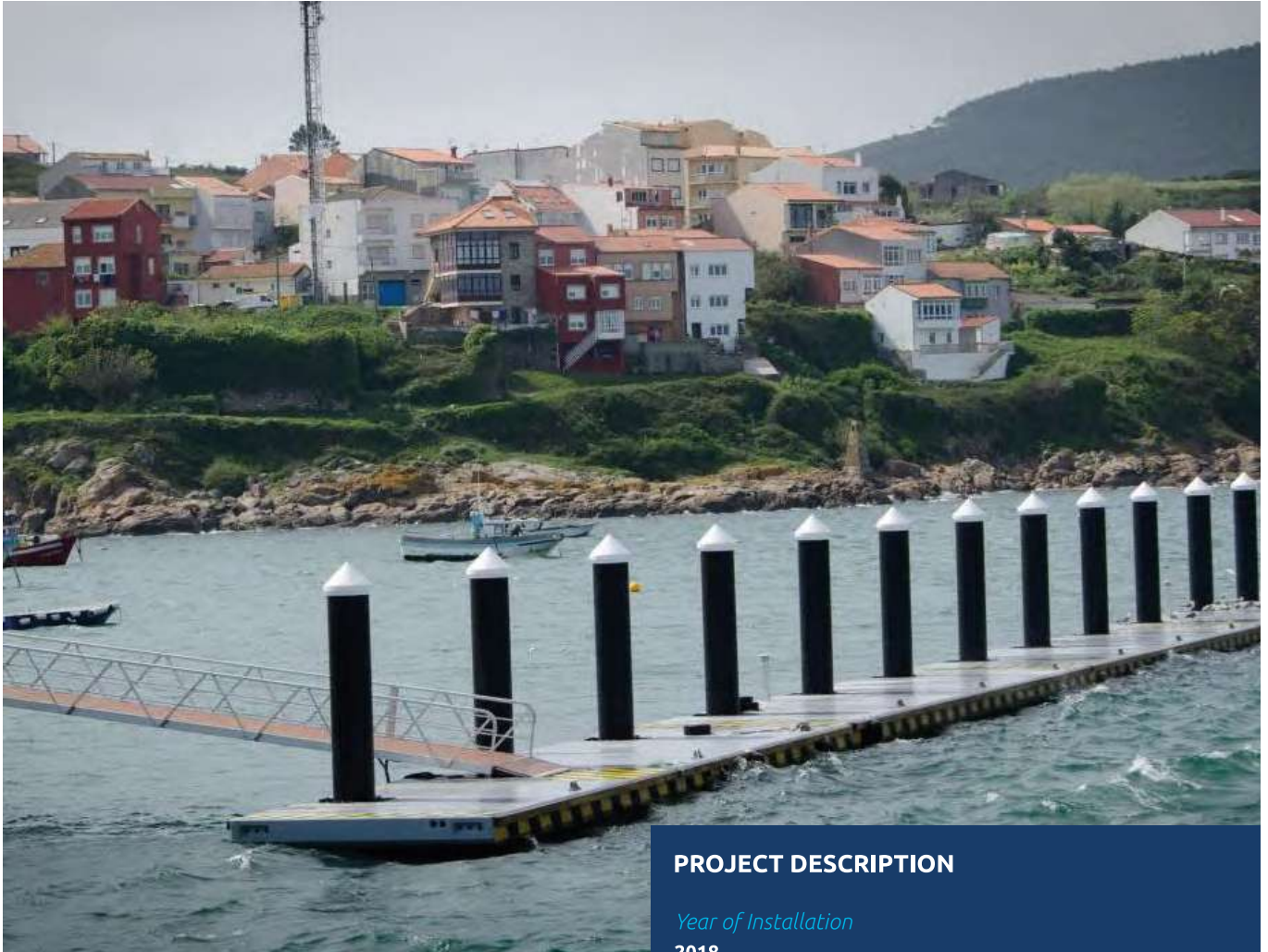
Piling works and installation provided by General Contractor.
